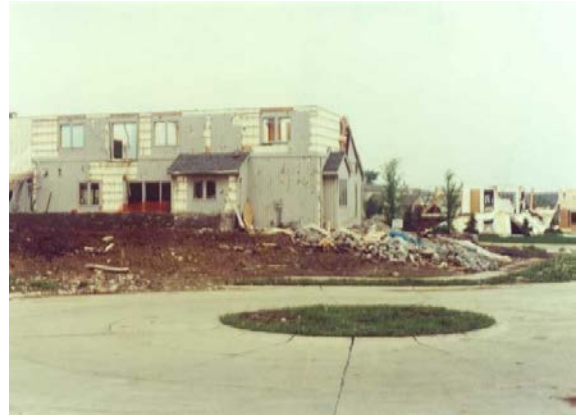
Figure 2: An ICF home survives a direct tornado strike with windows, siding, and roof destroyed.
